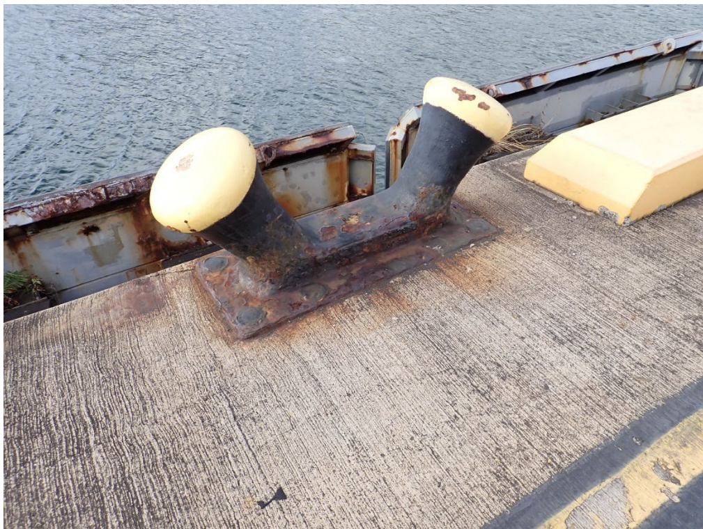
Photo 4: Typical Type B1/B2 Bollard
